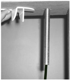
You will need a minimum 2" of clearance around nipple for white butterfly nut to attach.
