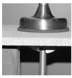
Tighten white butterfly nut onto threaded nipple until fixture is secure.
