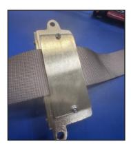
**STEP 6**Slide the tree strap so the buckle ends up on the opposite side of the jbox/fixture.
