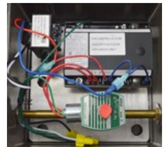
DBS997A1120V (120V) Direct Burial 9"x9"x7" Auto Ignition Control Box 120-Volt Option
