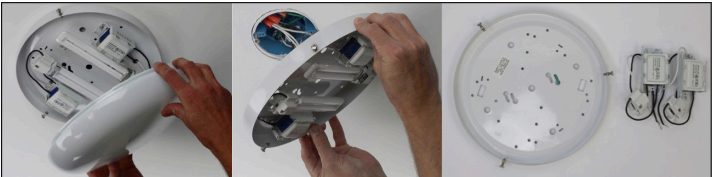
Remove Fixture & Disconnect Wiring
