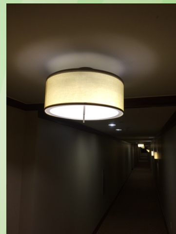
Focus Retrofit Install Is Identical In Color & Light Output With 25w Energy Savings Per Fixture
