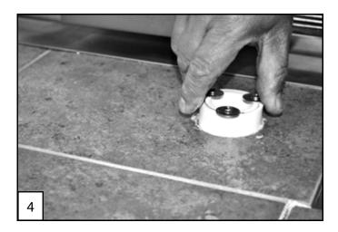
(4) Insert mounting sleeve into place. Rotate sleeve slightly to ensure even coverage of adhesive to sleeve. The washers will rest on the counter top holding the sleeve in place.
