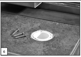
(6) After adhesive has completely cured remove the three #6 X 1" screws and washers. Keep screws for final assembly in step #8 and discard the washers..
