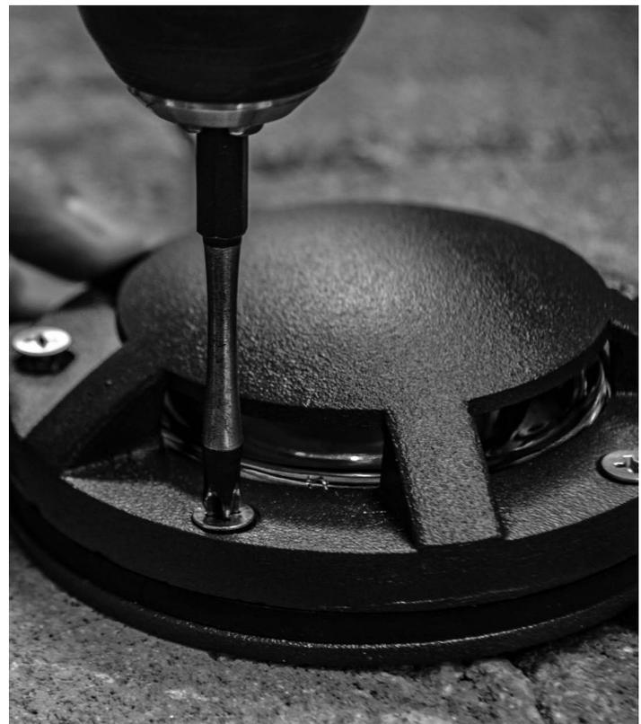
3. Insert anchor bolts into the two mounting holes
