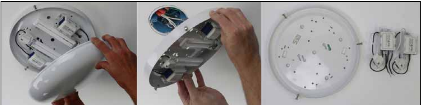
Remove Fixture & Disconnect Wiring
