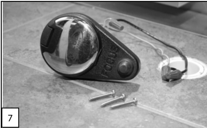
(7) Feed lead wire through mounting sleeve and make connection to 12v power supply.
