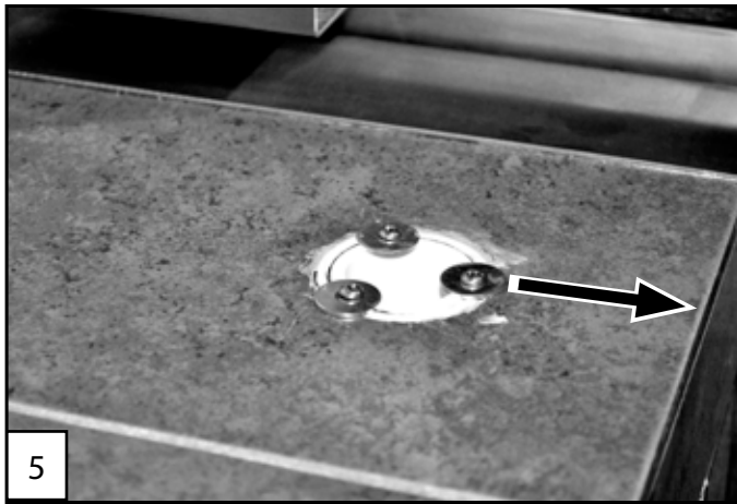
(5) Make sure to aim one of the screws towards the front of the counter. The front of the Quick Connect base will face this direction. Allow maximum drying time as specified by adhesive manufacturer.
