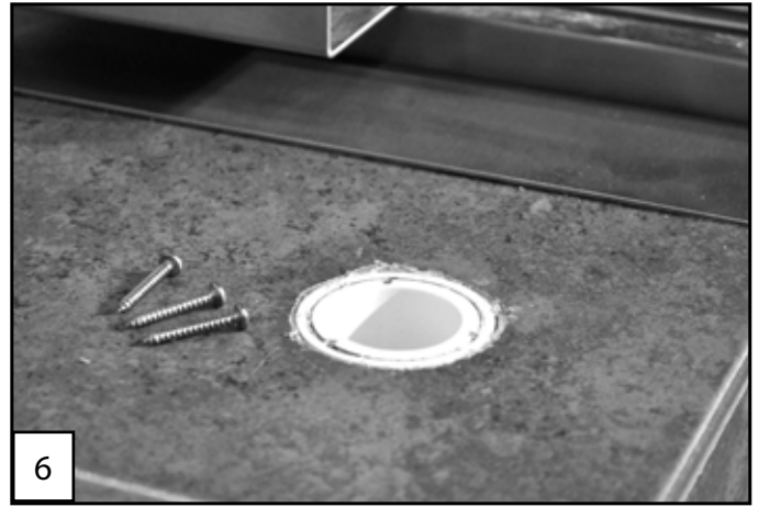
(6) After adhesive has completely cured remove the three #6 X 1" screws and washers. Keep screws for final assembly in step #8 and discard the washers..
