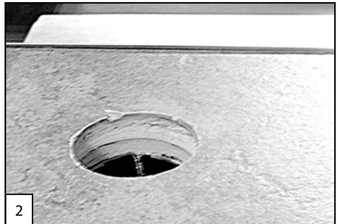
(2) Clean and dry hole prior to next step. Walls of hole should be free of dust, debris and moisture.
