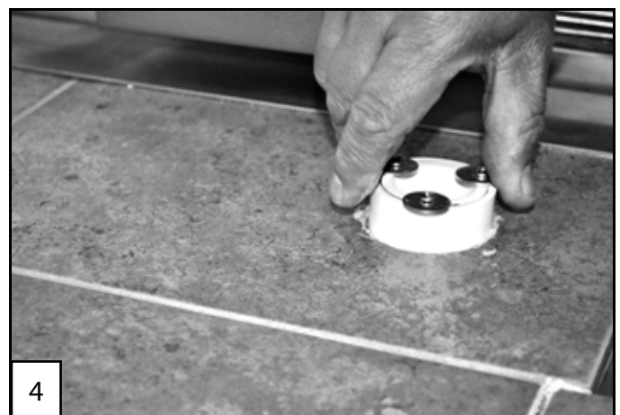
(4) Insert mounting sleeve into place. Rotate sleeve slightly to ensure even coverage of adhesive to sleeve. The washers will rest on the counter top holding the sleeve in place.
